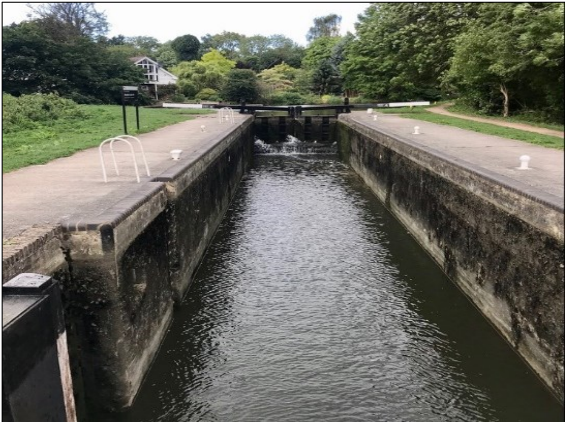
Figure 42 Hunsdon Lock near Hunsdon Mill
